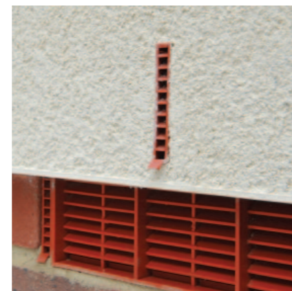
Cavity vents ensure the timber frame is kept dry. Here, the large vent is for a suspended timber ground floor.
