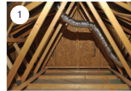
OSB sheathing on the gable wall
