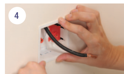
4 Position the box in the recess
