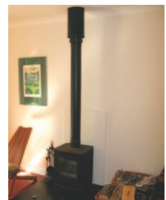
Careful positioning in relation to the timber structure simplifies the flue installation
