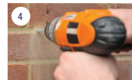
Begin removing bricks by drilling in the mortar
