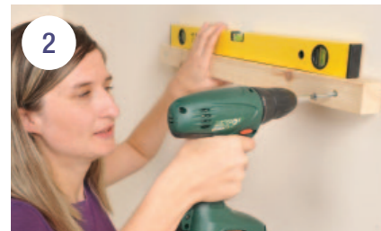
Level the batten then install the second screw
