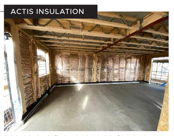
Actis insulation is a site fitted product that should be fitted when the structure is water tight.
