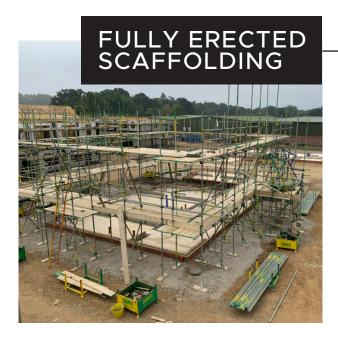
The agreed scaffolding should be fully wrapped around the slab prior to the timber frame starting.
