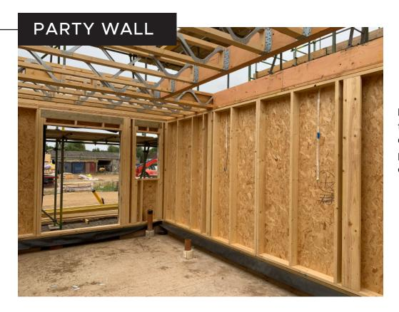
Fully sheathed party wall to EWT-2 robust detail. Contractor to insulate and plasterboard at a later date.
