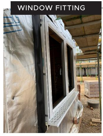
Windows should be fixed back to the timber frame. No requirements for window and door formers.
