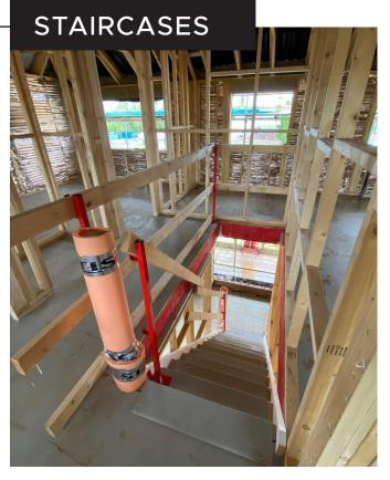
Staircases 1st fix completed. 2nd fix items such as handrails, balustrade will be supplied but fitted by the main contractor.
