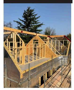
On occasions where we have room in roofs, we can construct the roofs with loose timbers and beams (cranked steels).
