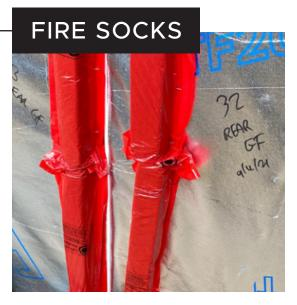
Cavity barriers are installed as part of the timber frame installation - a record is kept throughout the project.
