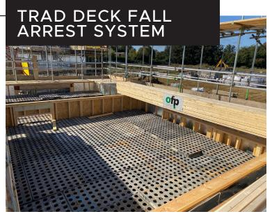
Trad Deck fall arrest safety system is the most common method of fall arrest prevention.
