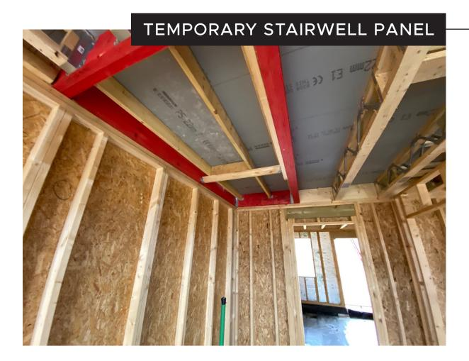
On completion of the floor joists and structural deck, all staircase openings should be fitted with a sacrificial temporary non structural floor panel - to be removed once the staircases are ready to be fitted.
