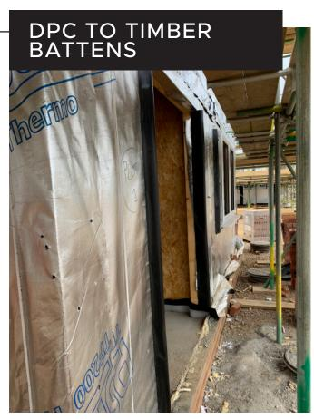
DPC must be also fitted to all window and door apertures prior to the brickwork contractor starting.
