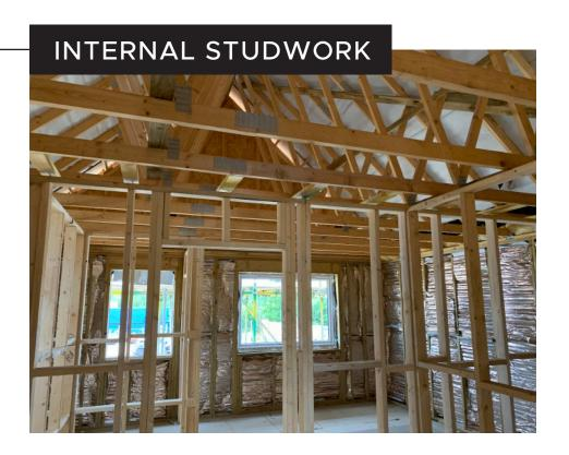
Non-load and load bearing Internal walls are constructed with 89mm CLS timber stud and come part of the timber frame package. They will be uninsulated and ready for 1st fix electrics and plumbing.
